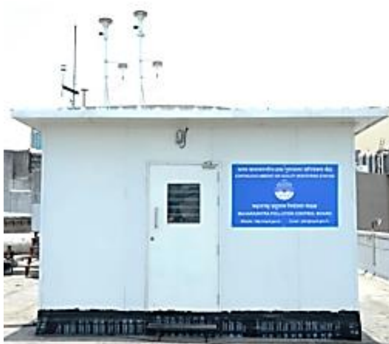
Continuous Ambient Air Quality Monitoring Stations at Kurla in Mumbai.
